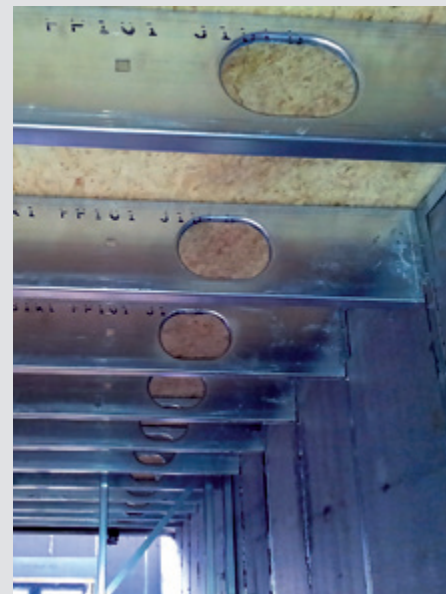
Large holes in light steel floor joists for integration of services
