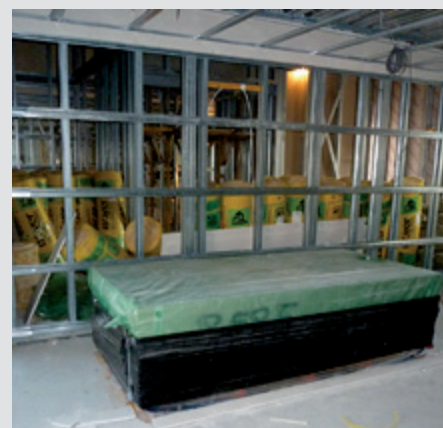
Construction materials stored on the floor of a light steel frame building
