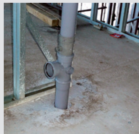
Individual opening for service pipe formed in a composite slab (maximum 150 mm diameter)
