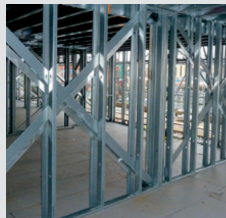
Cross-bracing in light steel frame walls forms a vital part of the frame stability
